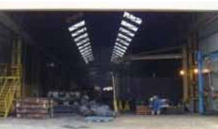
Bradken Foundry at Ipswich saves $10,000 a year by installing skylights.
