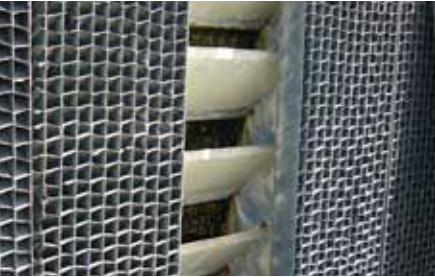
Installing drift eliminators promotes air circulation and reduces drift losses.
