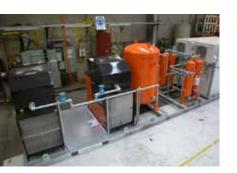
Compressor system consisting of (left to right) a nitrogen generator used for food packaging, four air filters, a receiver tank and two compressors.
