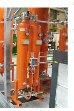
Air compressor filters should be kept clean to reduce pressure drops.
