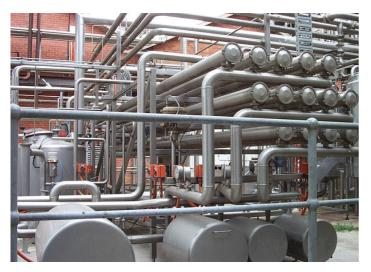
Membrane filtration is a higher level treatment that recovers product or removes unwanted components. This improves the quality of the permeate increasing the possibilities for reuse within the plant.
