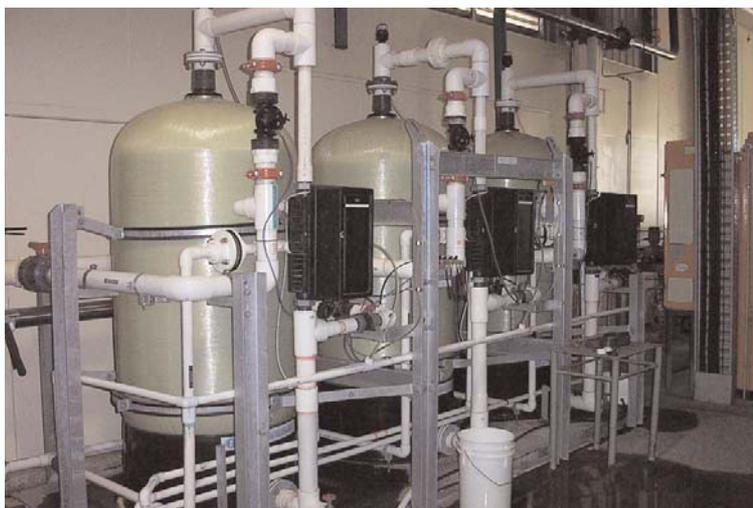
*The treatment of boiler feedwater will help to minimise build-up of scale, which acts as an insulator and inhibits heat transfer.*
