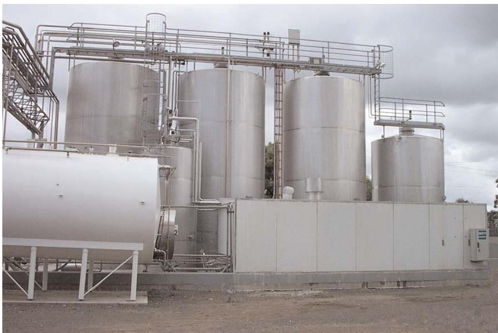
*The main advantage of multi-use CIP systems is that they can recirculate and allow the reuse of chemicals and rinse water, thereby substantially reducing water and chemical consumption.*
