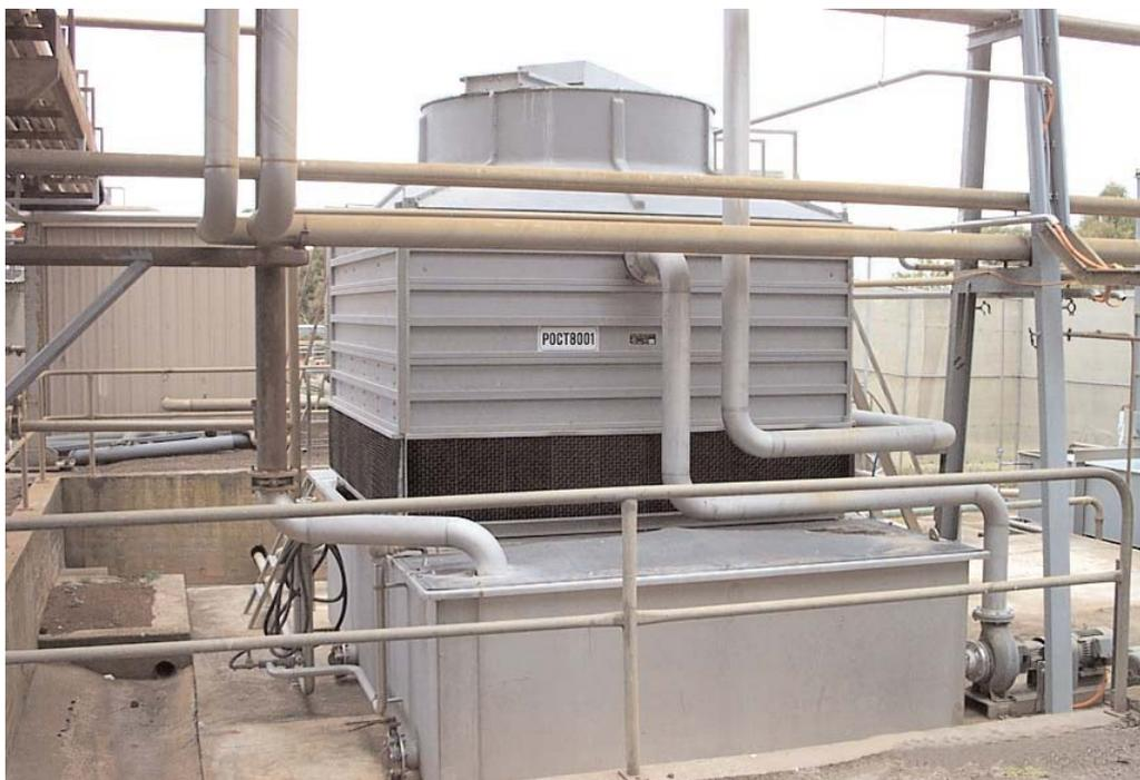
*Cooling towers should be regularly checked for leaks and scale build-up.*
