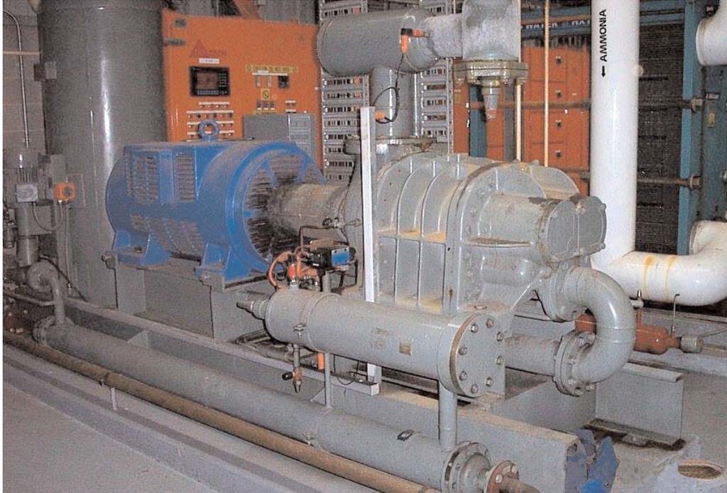
*The compressor is the workhorse of a refrigeration system and usually accounts for between 80% and 100% of the system's total energy consumption.*
