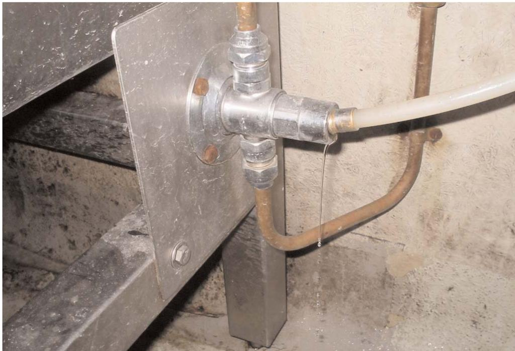
*Taking supply water meter readings during non-production hours can highlight any unusual water consumption or leaking pipes.*
