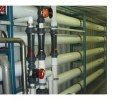
Water treatment systems generally use UF or MF as a pretreatment system prior to RO. RO is often used to polish water rather than remove larger molecules. Pretreatment reduces membrane fouling and backwash requirements.
