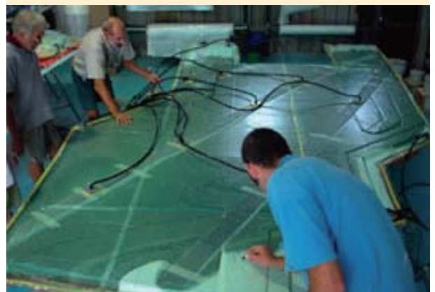
Reinforcement materials are sealed with a membrane until airtight
