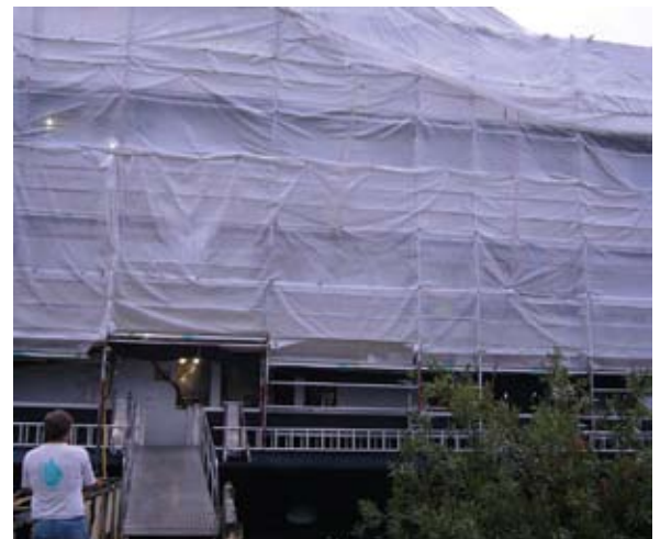
Working on water with protective sheeting in place
