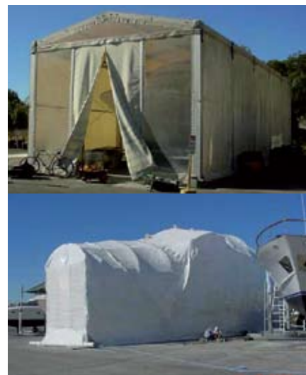
Examples of suitable enclosures for spray painting and abrasive blasting in the open
