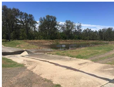
Figure 3: First flush pond with overflow (Courtesy of TEYS Beenleigh)
