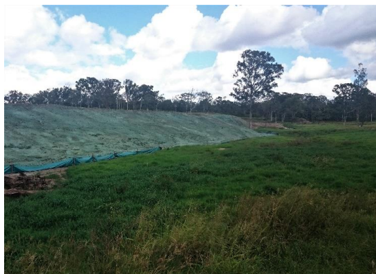
Figure 16: Hydro-mulching
