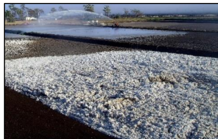
Foaming on crusted anaerobic ponds
