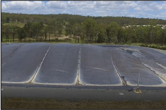
Covered Anaerobic Lagoon or CAL Image: Teys, Beenleigh
