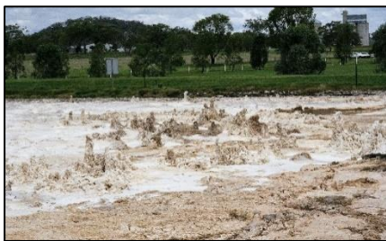
Gas geysers on crusted anaerobic ponds Image: Courtesy of Johns Environmental
