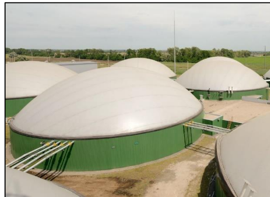
Mixed Vessel Anaerobic Reactor
