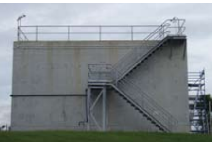
UASB at Foster's Australia
