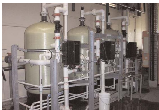
The treatment of boiler feedwater will help to minimise build-up of scale, which acts as an insulator and inhibits heat transfer.
