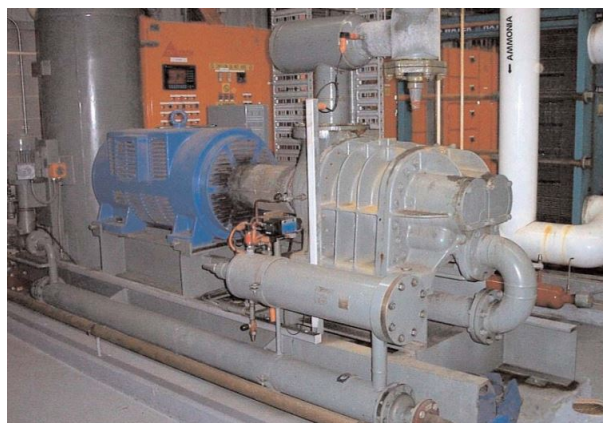
The compressor is the workhorse of a refrigeration system and usually accounts for between 80% and 100% of the system's total energy consumption
